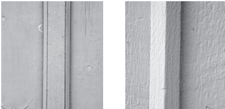
Battens: A typical flat batten on the left; on the right, a Patterson “beveled” batten.
