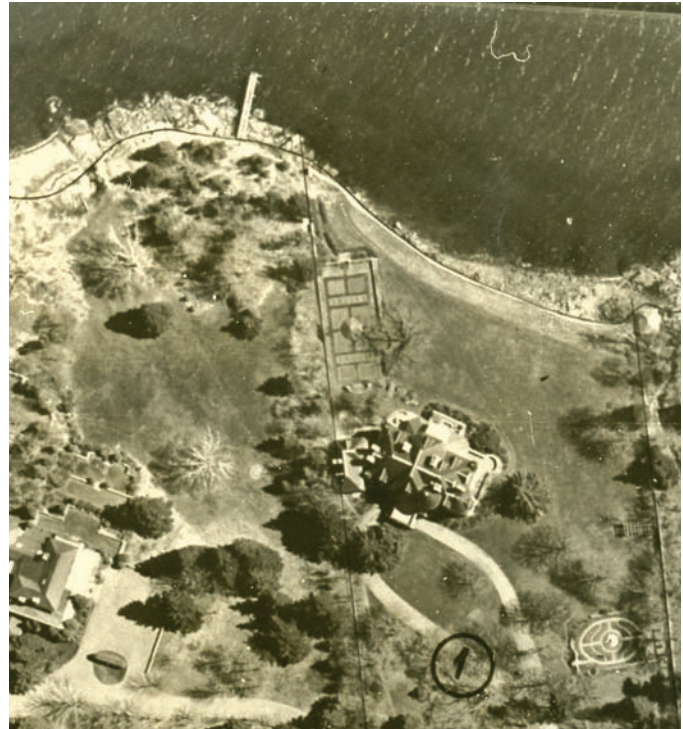
Aerial photograph of The Turrets (center) and the Sunken Garden (lower right). Photographer unknown, ca. 1950. Courtesy of College of the Atlantic Archives Photograph Collection
