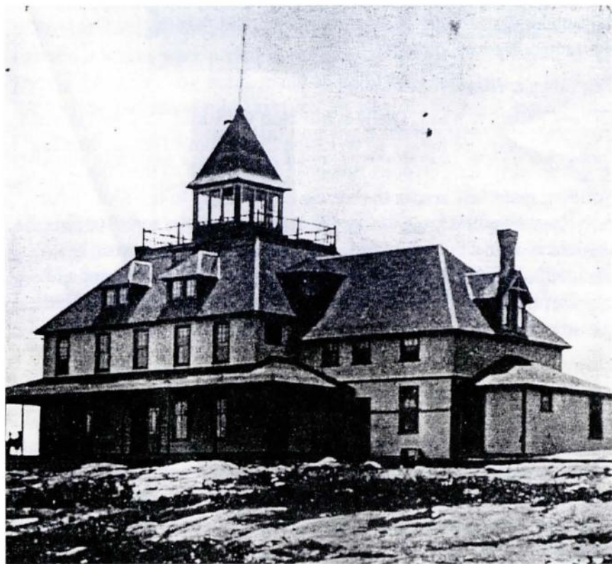
The Green Mountain House was built in 1883. The following summer, sparks from the kitchen chimney (right) ignited a section of the main roof and the entire "structure" burned to the ground.
