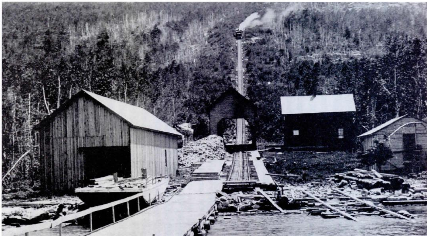
The Green Mountain Railway track began at the east shore of Eagle Lake and stretched 6,300 feet up Green Mountain's west slope. The course was nearly straight and gained 1,258 feet in elevation between the lakeshore and the summit.
