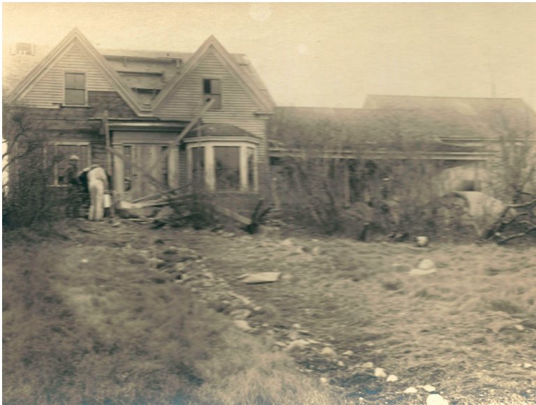
Four Winds during its restoration, 1928. Courtesy of the author
