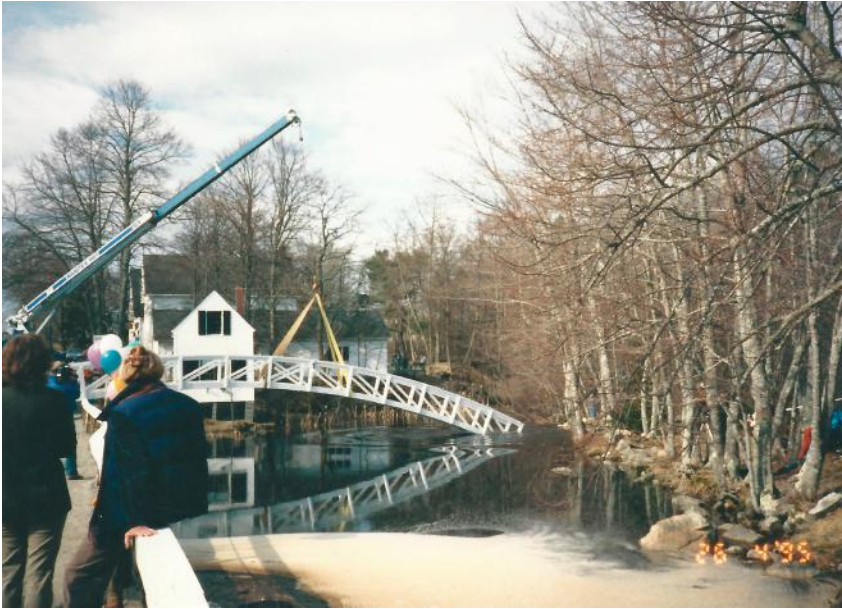
A replacement bridge, built with pressure-treated lumber, is installed in 1995. Mount Desert Island Historical Society
